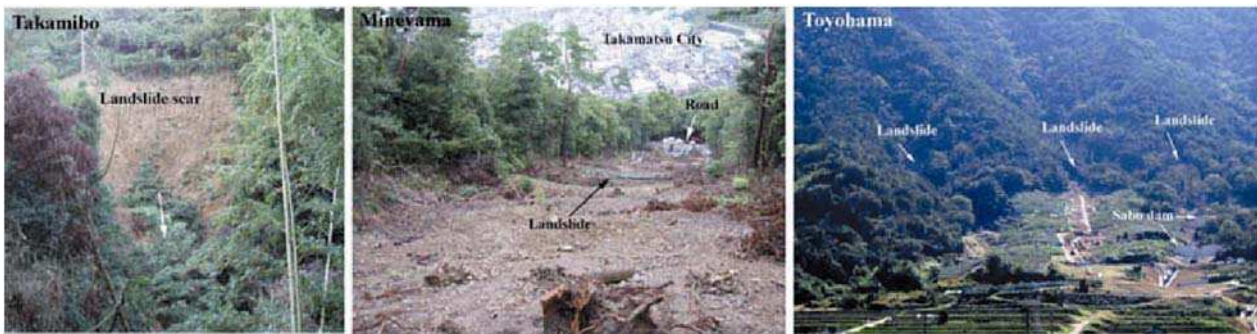
Figure 11. Rainfall triggered flow-like landslide in Kagawa (Takamibo, Mineyama and Toyohama)
